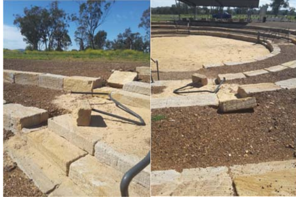
The damage caused by vandalism in the amphitheater at the Myall Creek Memorial.
