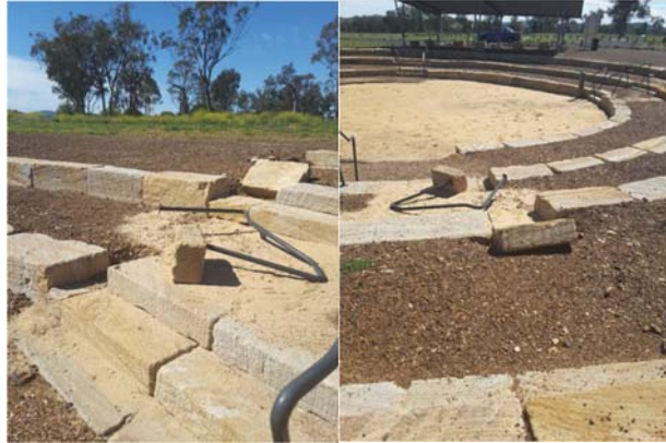
The damage caused by vandalism in the amphitheater at the Myall Creek Memorial.
