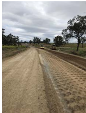
Stabilising the sub-base of the 1.3km section of RR7705 North Star Road.
