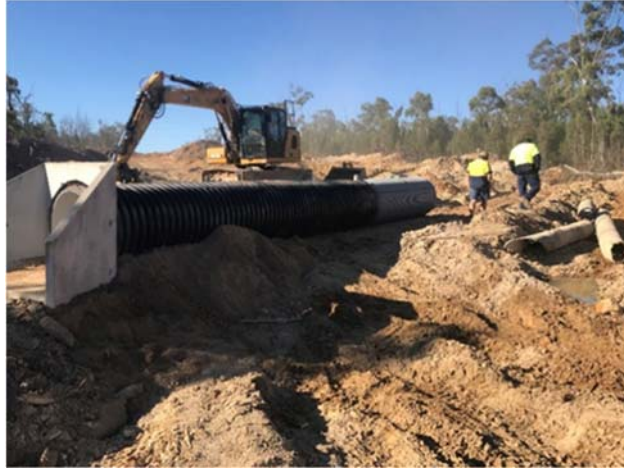
Installing new pipes on the HPV Route.
