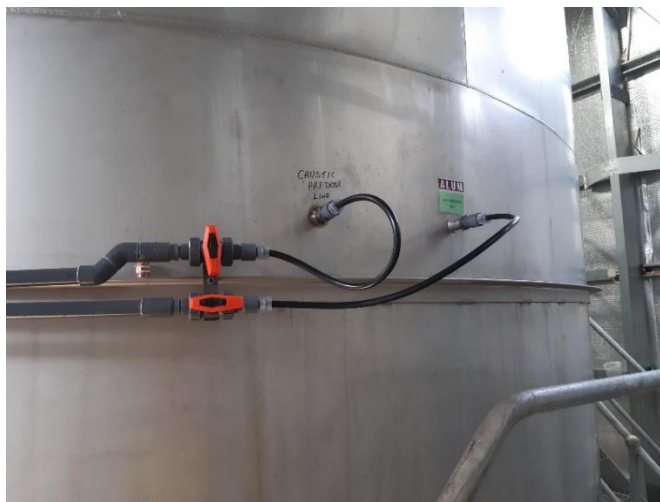
Bingara water treatment plant dosing line modifications
