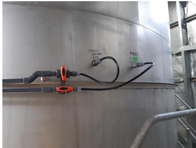
Bingara water treatment plant dosing line modifications
