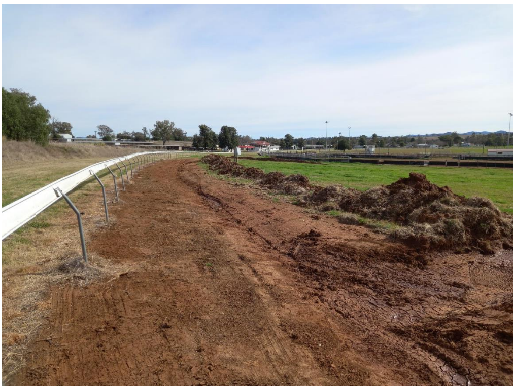
Bingara showground track drainage
