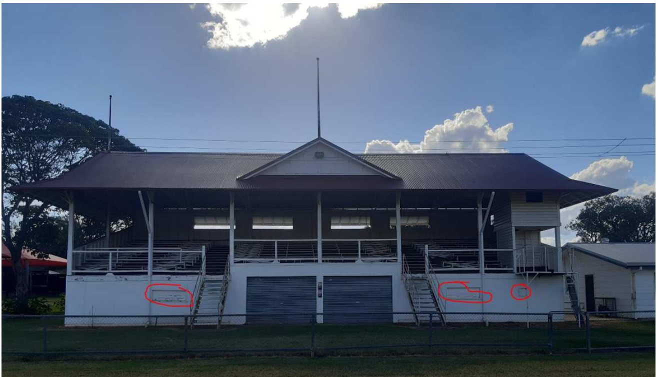
Front of grandstand showing windows to be sheeted over
