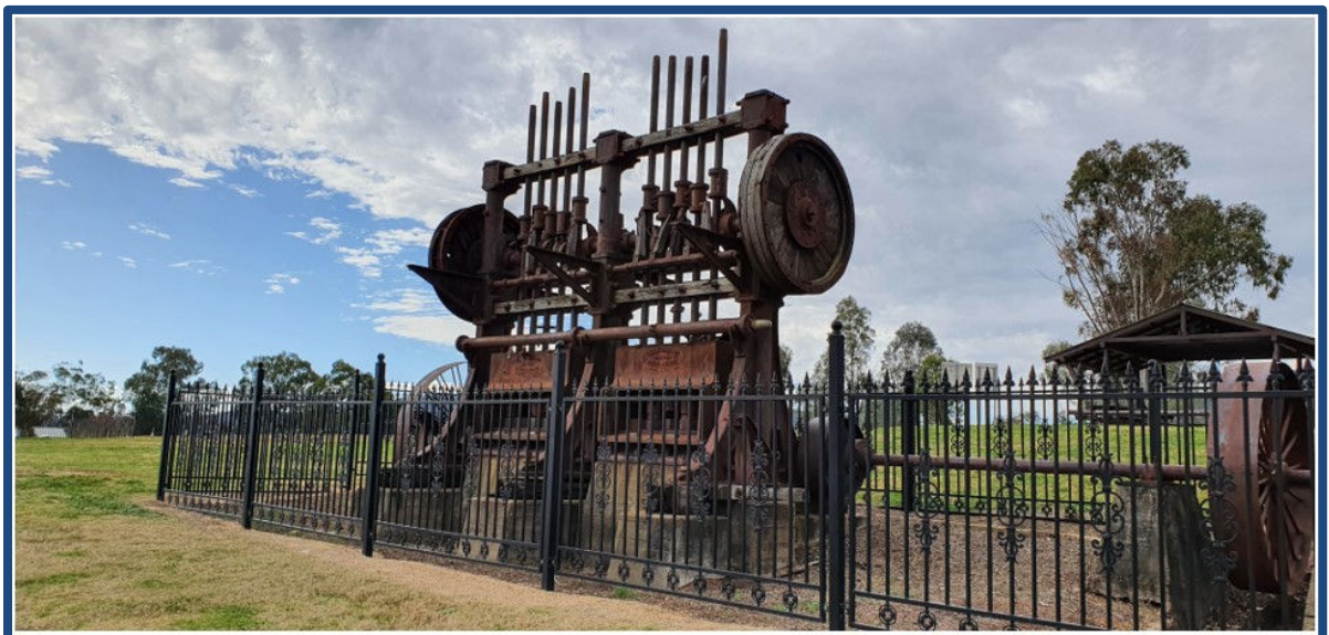
Figure 13 - Assets Metal enclosure fencing erected on the perimeter of the Stamper Battery site.
