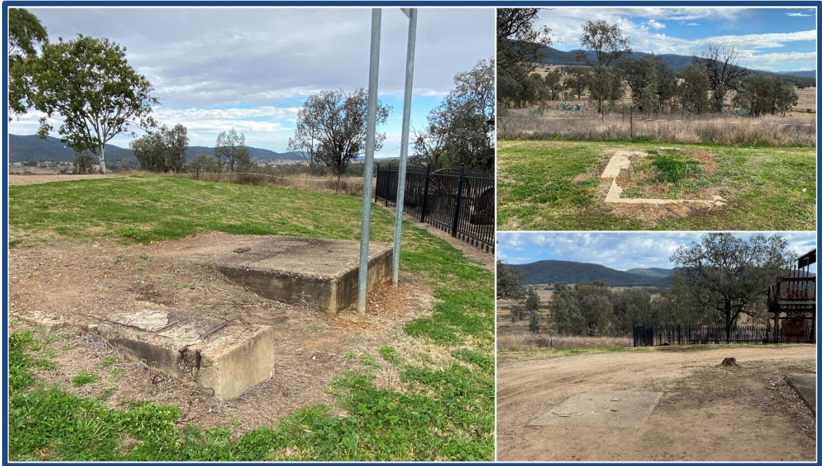
Figure 17 - Assets Various concrete mine shaft cappings or pads for infrastructure demonstrate the history of mining at All Nations Hill.
