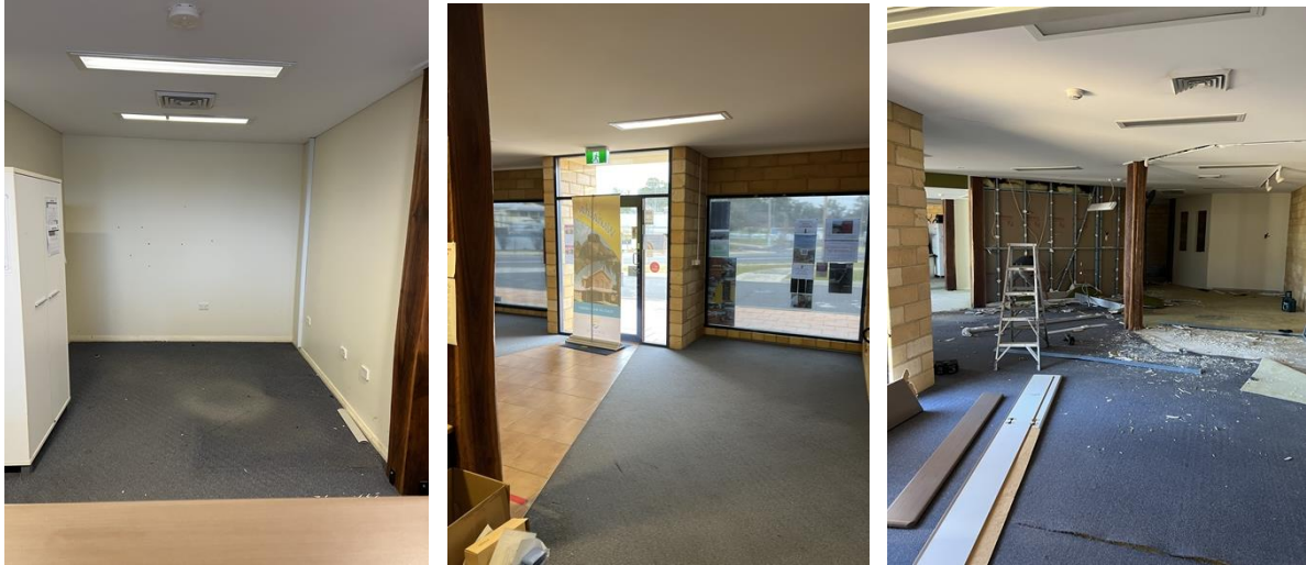
Warialda Visitor Information Centre Renovations
