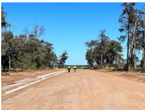
SR9 IB Bore Road
