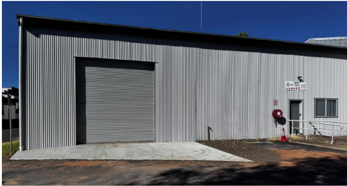
Warialda RFS Fire Control Centre
