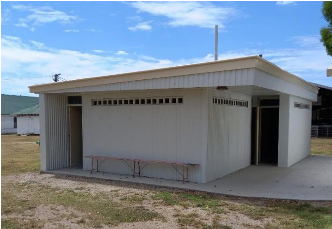
Exterior has been painted and new concrete paths surrounding the amenities block
