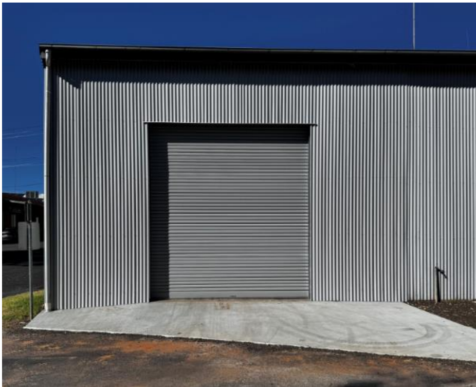
Old loading dock removed and new roller door installed
