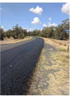
cement/flyash blend) is spread at a rate of 2.5% over the patch. Council's Asphalt Zipper is then used to mill and incorporate the existing soil with the additive, adding moisture and then re-compacting to form a new pavement. Once compacted, the patch is sealed with a double coat 7 mm emulsion seal using Council's Jetpatcher and the line marking is reinstated where required. This year only saw 2,120 m<sup>2</sup> of heavy patching completed on MR063 Fossickers Way.
