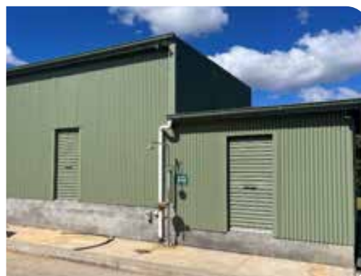
Northern wall at Bingara water treatment plant
