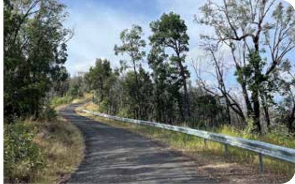
Batterham's Lookout guardrail
