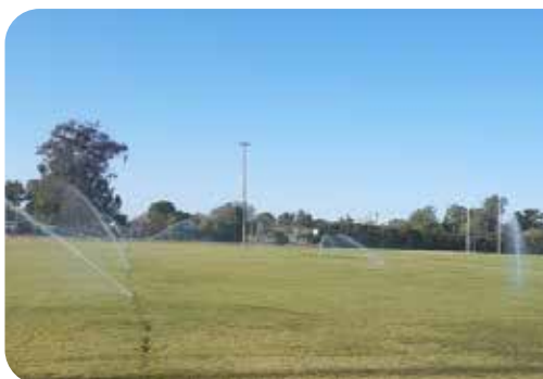
No 2 Oval underground irrigation
