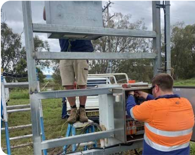
Gravesend switchboard replacement
