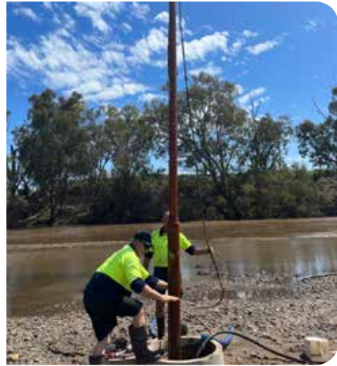
Gravesend bore replacement
