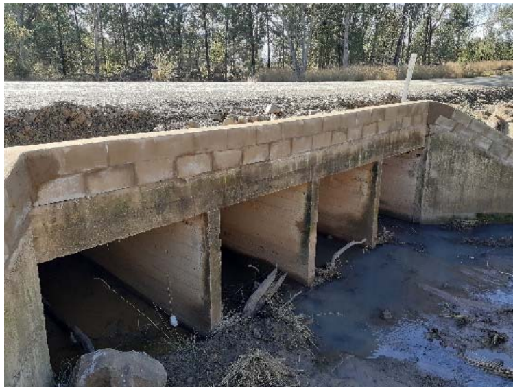
Headwall raised on SR11 Horton Road.
