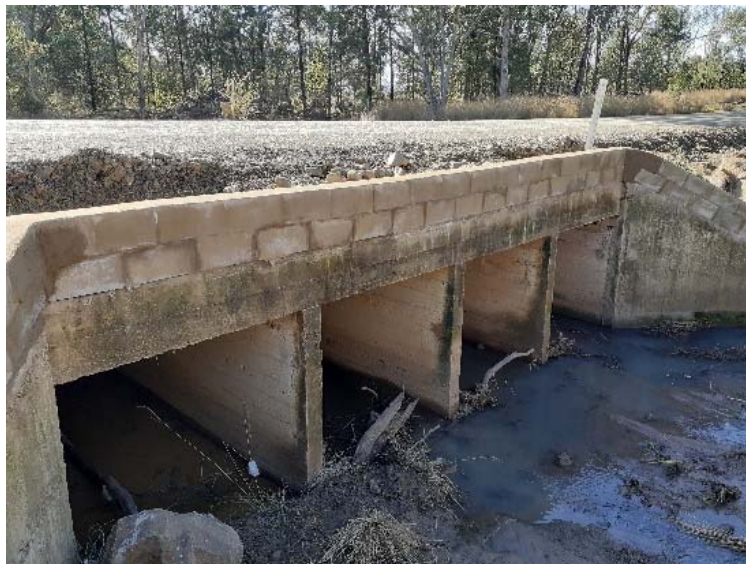
Headwall raised on SR11 Horton Road.
