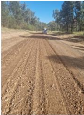
Oregon Road Maintenance Grade with Polycom Addition
