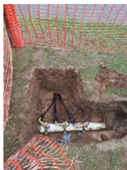
Under-bored Service Lines in Bombelli Street
