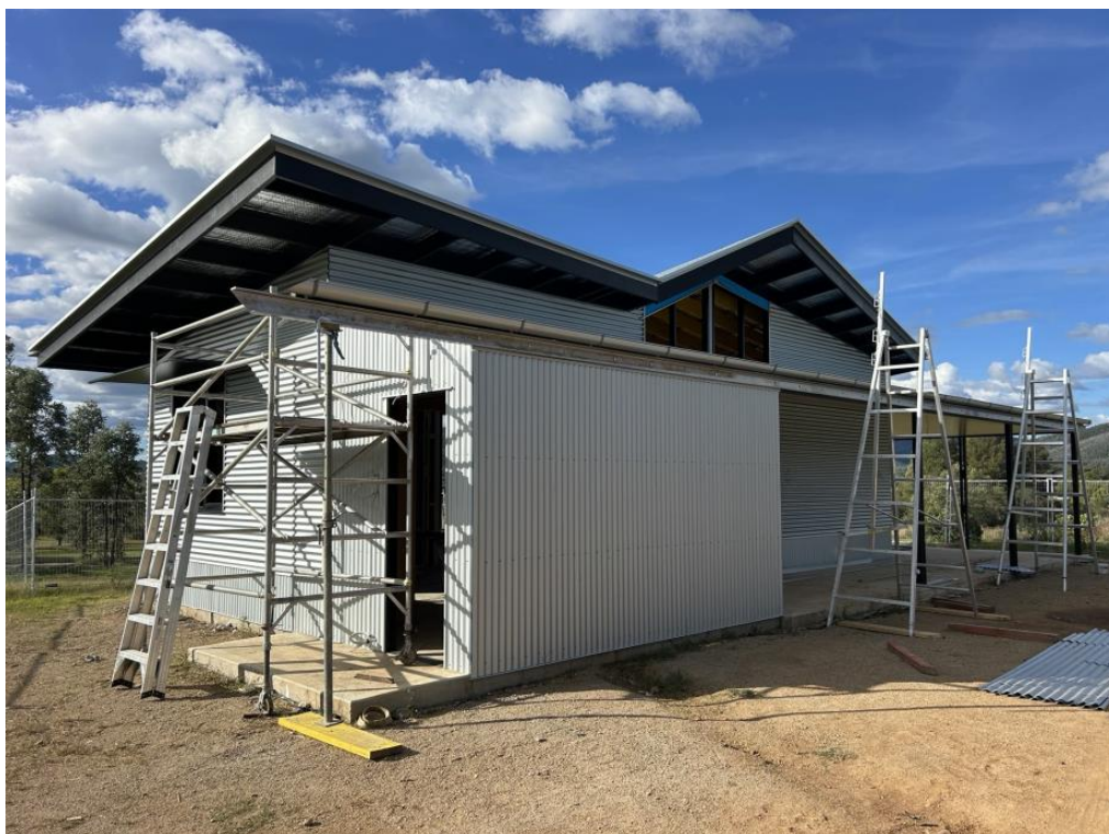
External cladding of the common room
