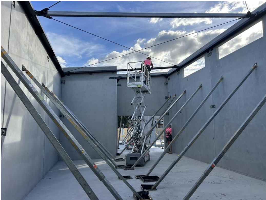
Erection of structural steelwork within Council Chambers
