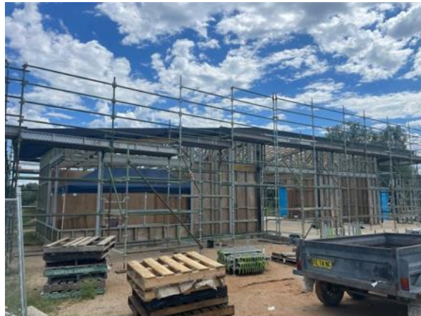
Scaffolding installed for roofing works
