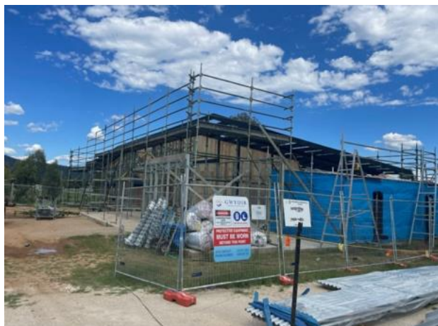
Scaffolding installed around main building
