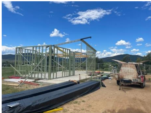
Common Room – framing completed
