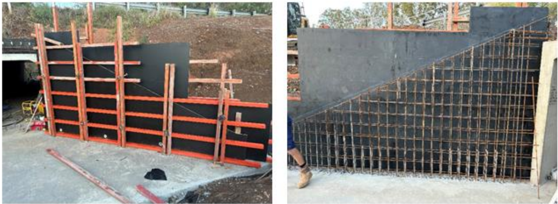
Preparation of box culvert wingwalls and steel at the Wendouree Rehab site.
