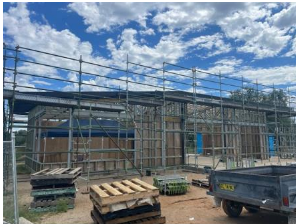
Scaffolding installed for roofing works
