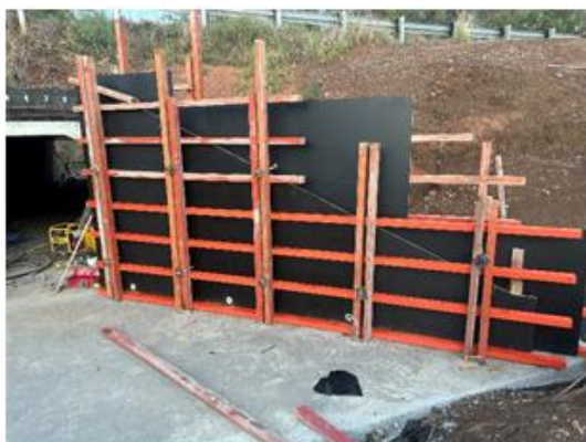
Preparation of box culvert wingwalls and steel at the Wendouree Rehab site.
