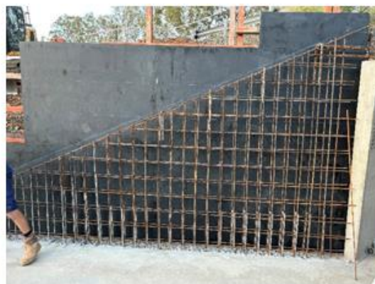
Preparation of box culvert wingwalls and steel at the Wendouree Rehab site.
