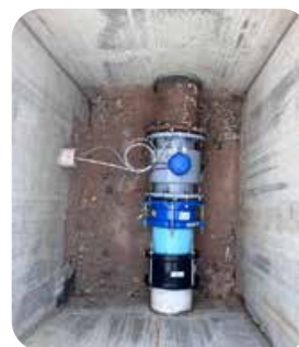
Warialda South Reservoir outlet meter
