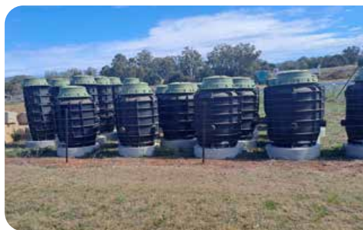
Pressure sewer pump stations
