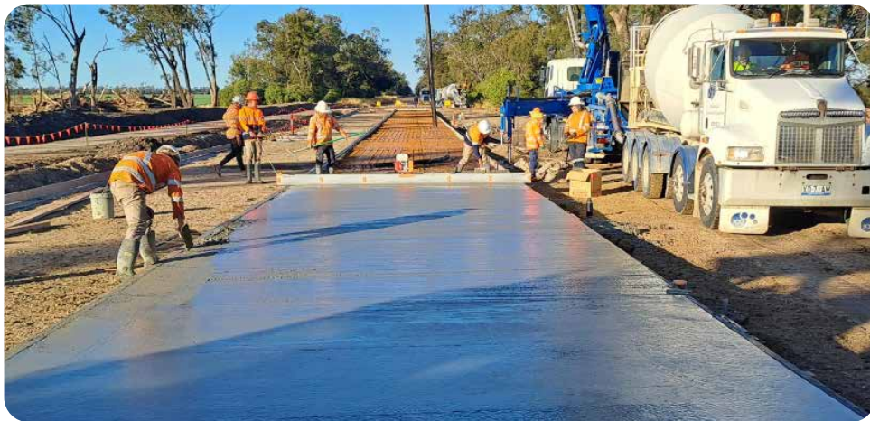
County Boundary Road Floodway 6 – placement of concrete on the western side of the new causeway.
