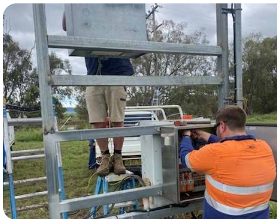
Gravesend switchboard replacement
