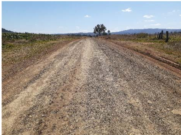
Gravel resheeting SR11 Horton Road flood damage.
