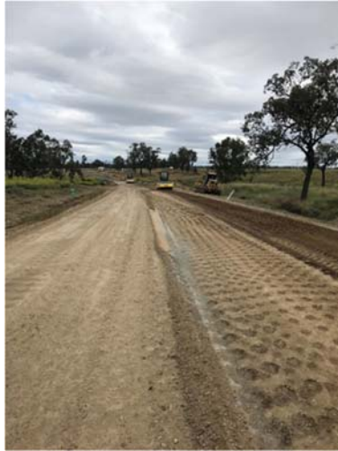
Stabilising the sub-base of the 1.3km section of RR7705 North Star Road.
