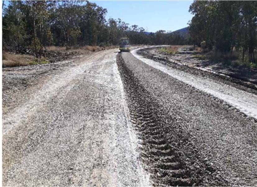
The upgraded pavement being stabilised on SR11 Horton Road.
