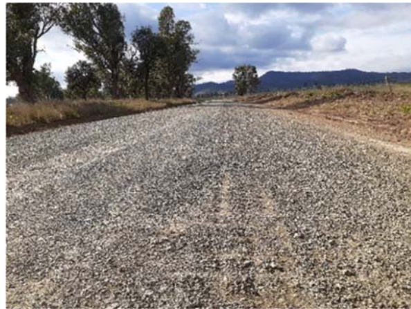
Gravel resheeting SR11 Horton Road flood damage.
