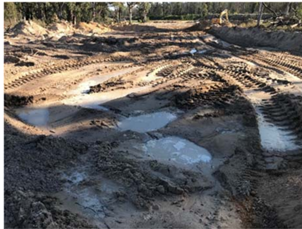
Unsuitable sand material being removed from the HPV Route.
