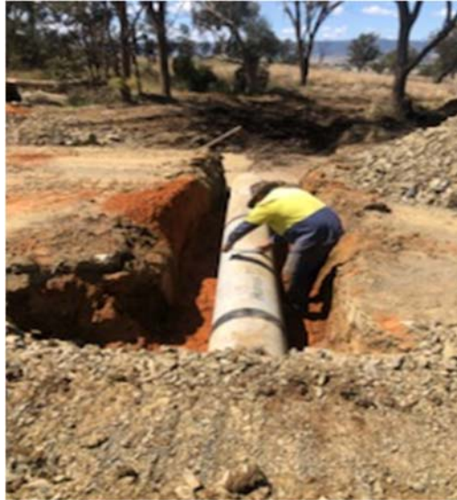
New 450mm pipe being installed ahead of construction crew on SR11 Horton Road.
