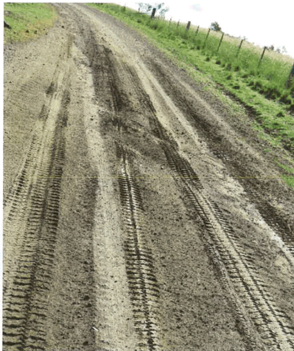
Figure 4: Figures 2,3 and 4 show the poor condition of the road in "Glen Owen" which is to be resheeted before June 2020
