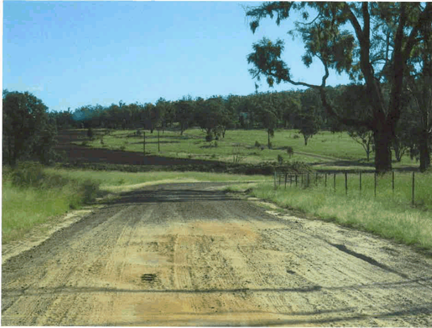
Figure 5: Badly degraded section of the schoolbus route
