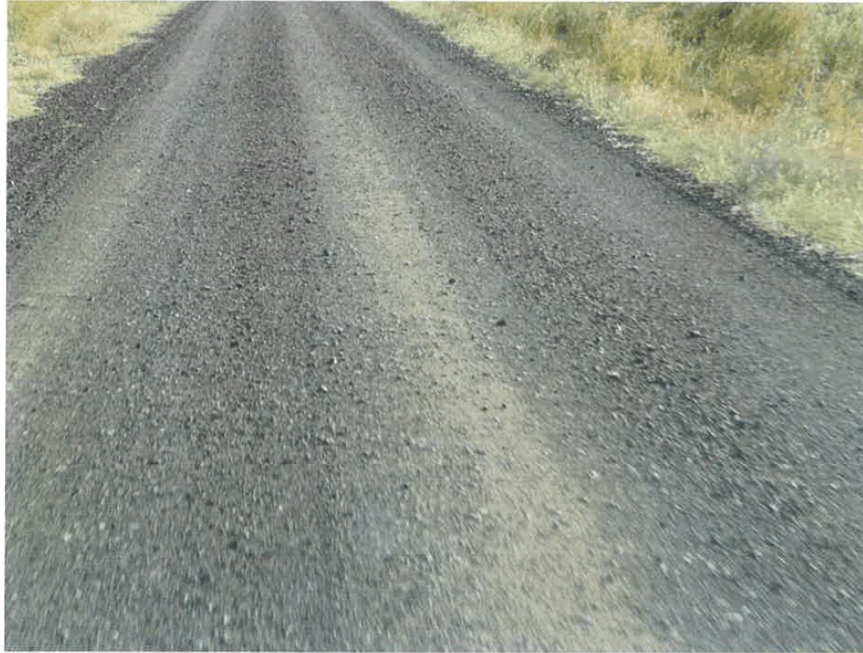
Figure 2: Part of the resheeted section of road which has stood up to local traffic with virtually no maintenance
